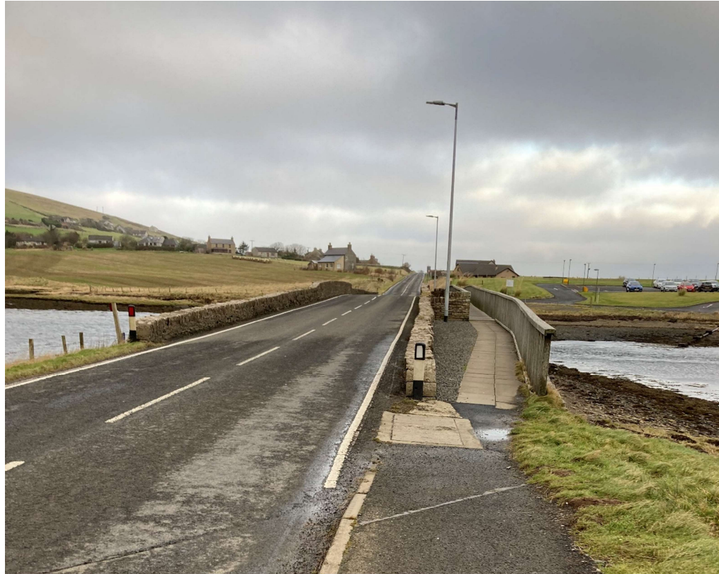
Figure 10. Ouse Pedestrian Bridge
