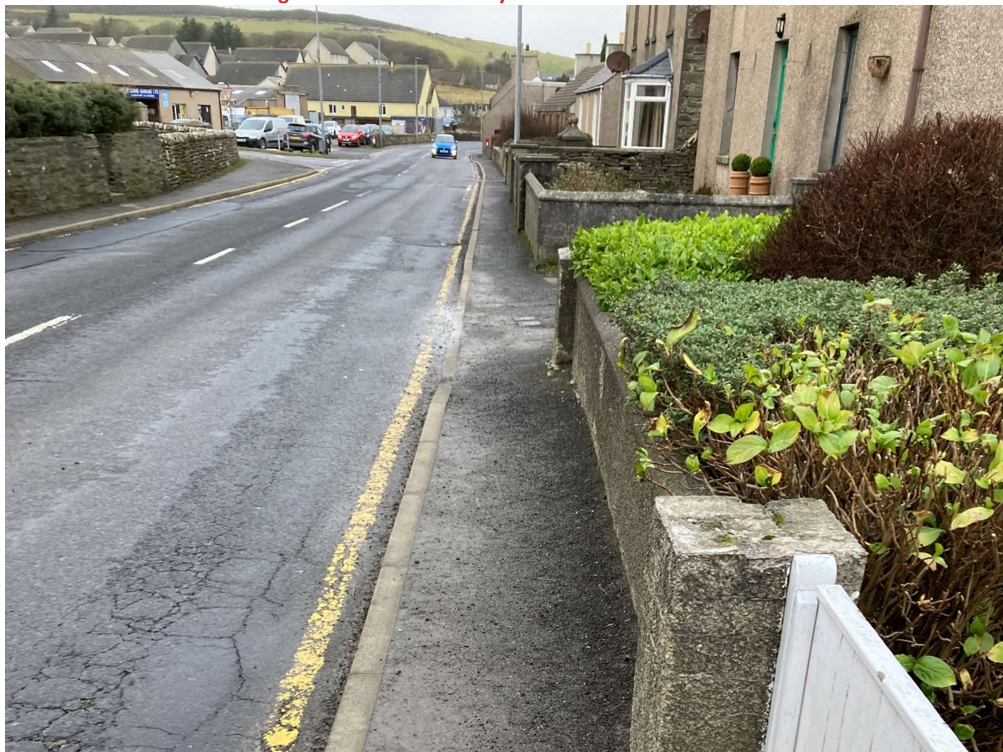
Figure 3. Narrow Footways on A965
