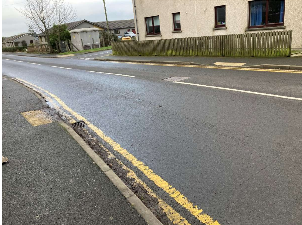
Figure 5. Uncontrolled Crossing Facilities at A965/A966 Junction
