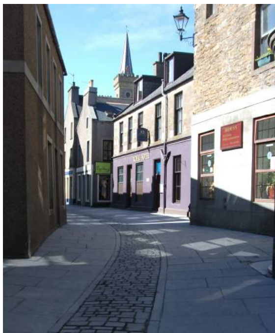
Above Fig. 22 Shared surface street Stromness
