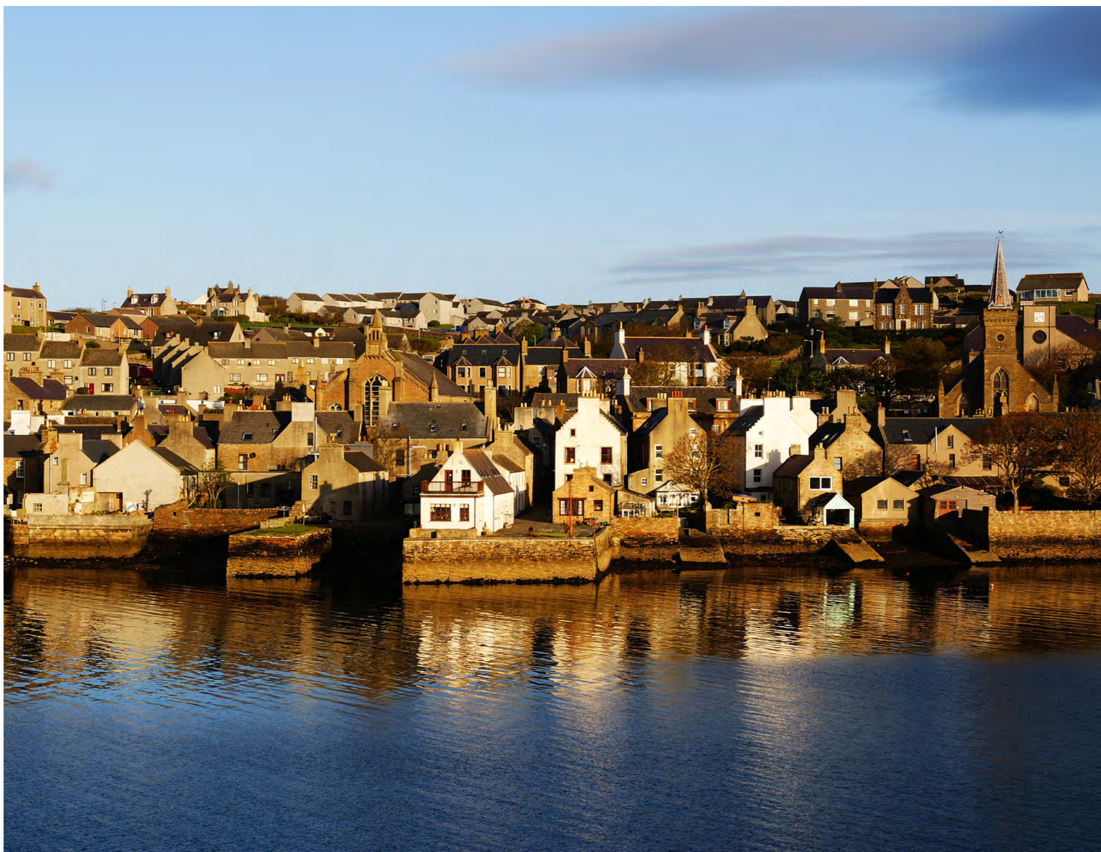
View of the historic piers and skyline of Stromness
