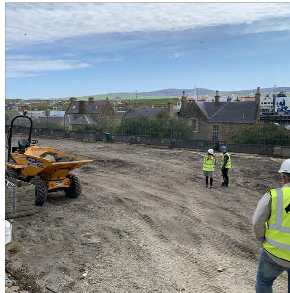
View from old primary school site - June 2019
