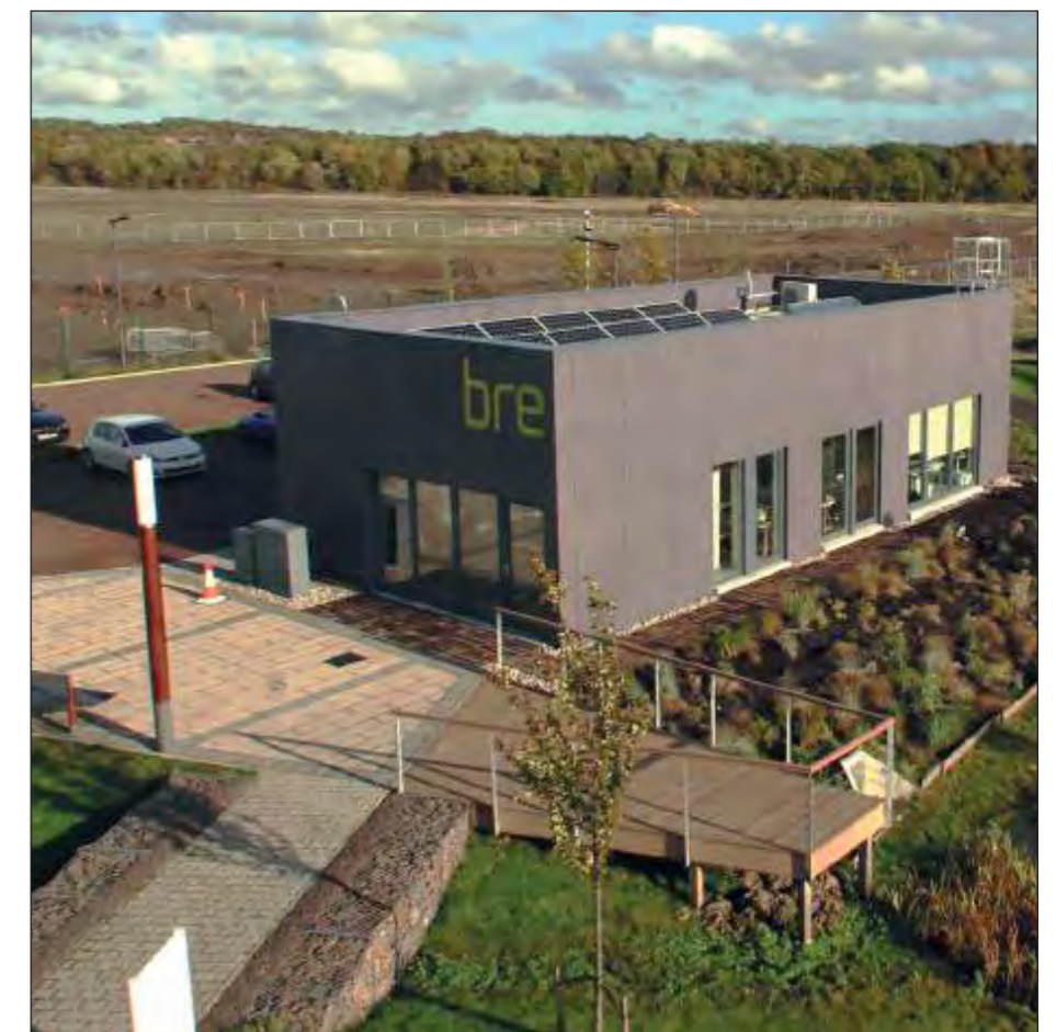
Image of precedent project, BRE Ravenscraig interpretation centre - passive design & pre-fabricated unit
