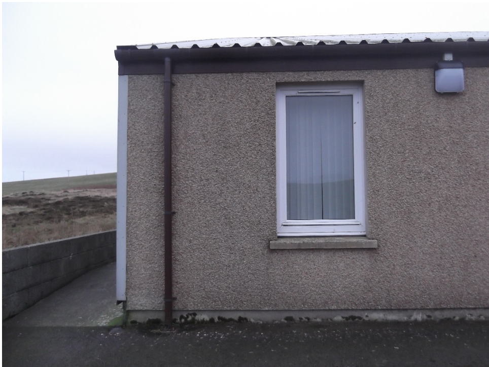
Area of hall at the front where the vehicle charge point will be located.
