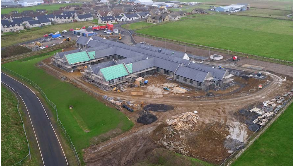
Hamnavoe House, Stromness under construction.
