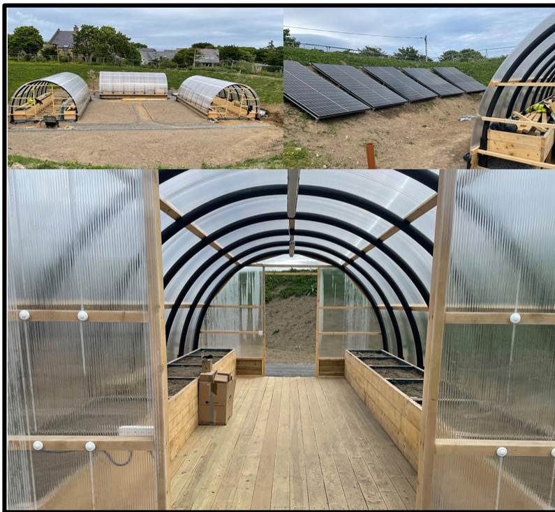
Figure 3.7: Polytunnel build progress, solar panels and internal structure.
