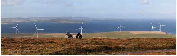
Turbine Tip Height: 149.9 m Hub Height: 82 m Rotor Diameter: 136 m
