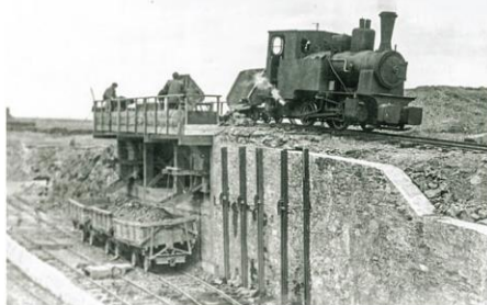
The stone crushing plant near Housebreck Quarry, Burray. June 1943
