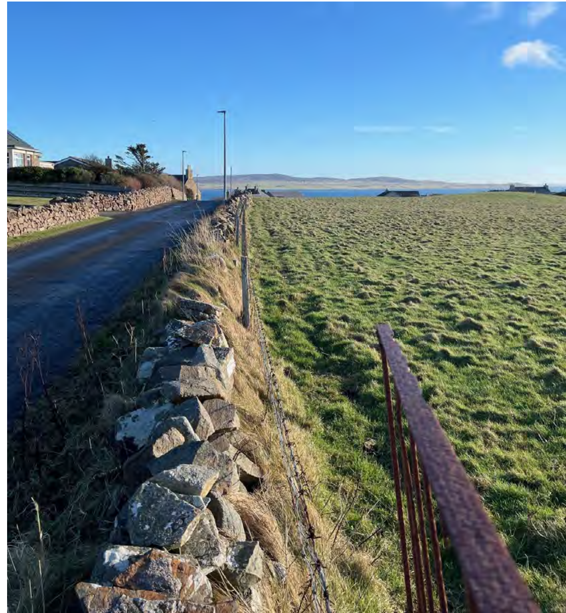
Figure 31: Drystone Dyke boundary along Outertown Road of STR-16
