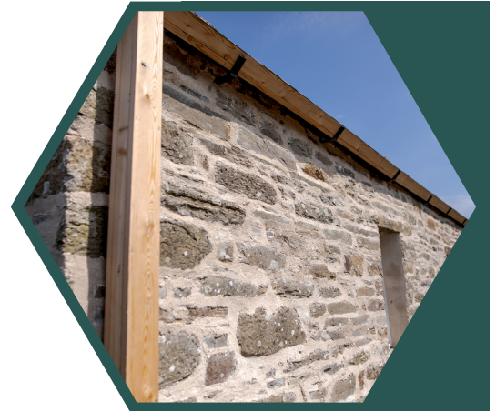
New pointing and guttering
