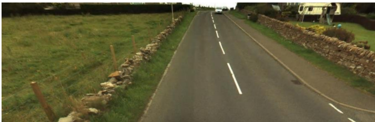
Site area – note narrow width of the verge, well below 1.8m wide and note safe and well maintained footpath opposite to which the site can connect
