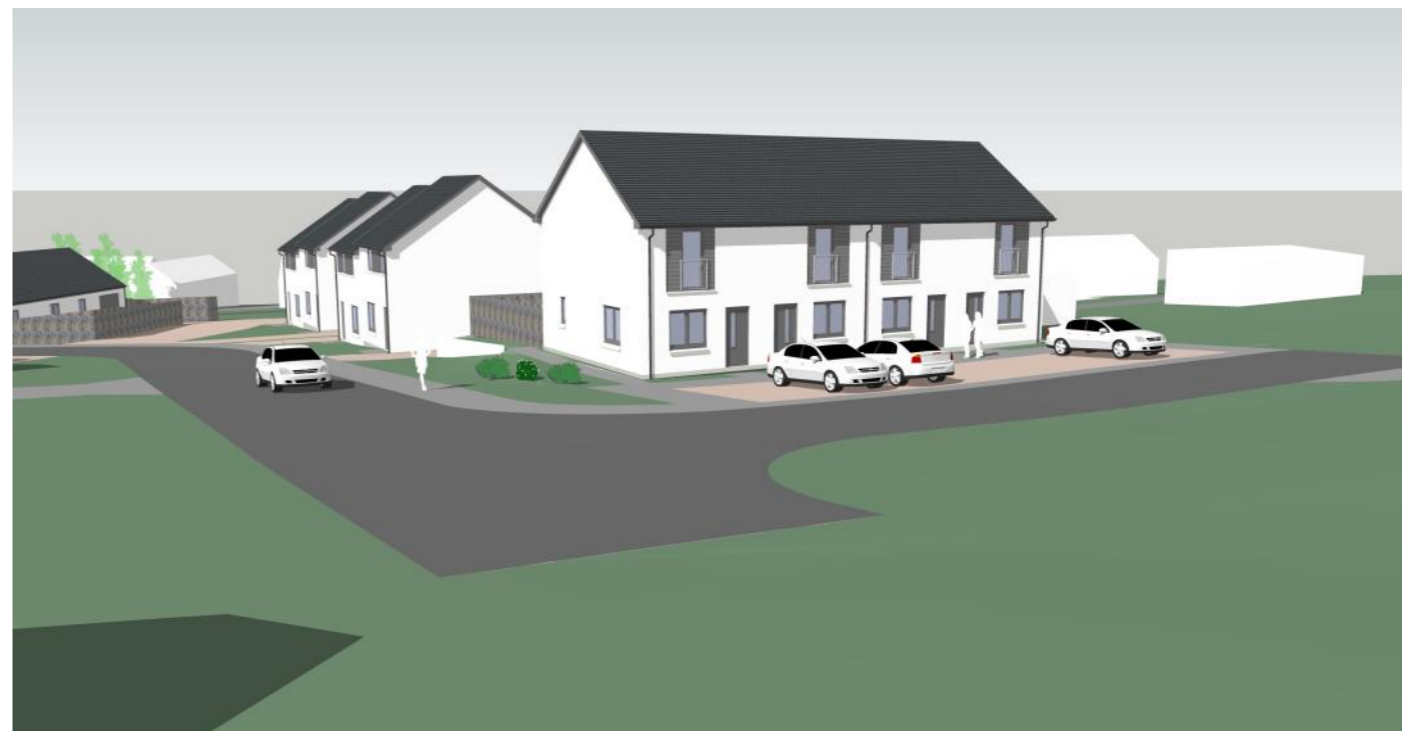
VIEW OF TERRACED BLOCK LOOKING SOUTH-WEST
