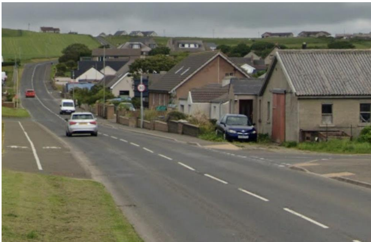
Cairston Road and existing footway running along the south side of the road
