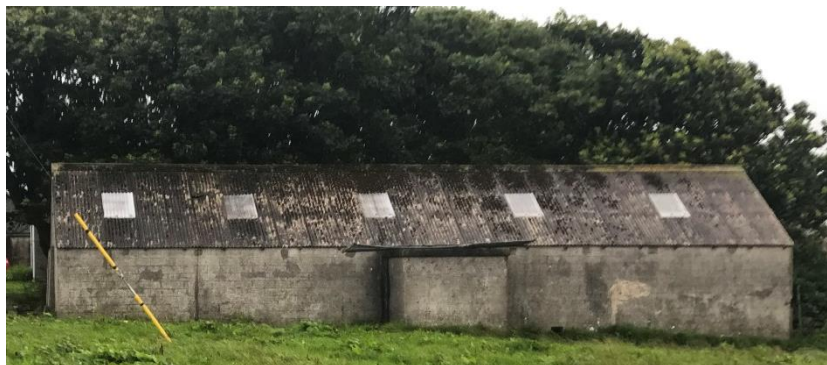
Agricultural Buildings at C as viewed from the field
