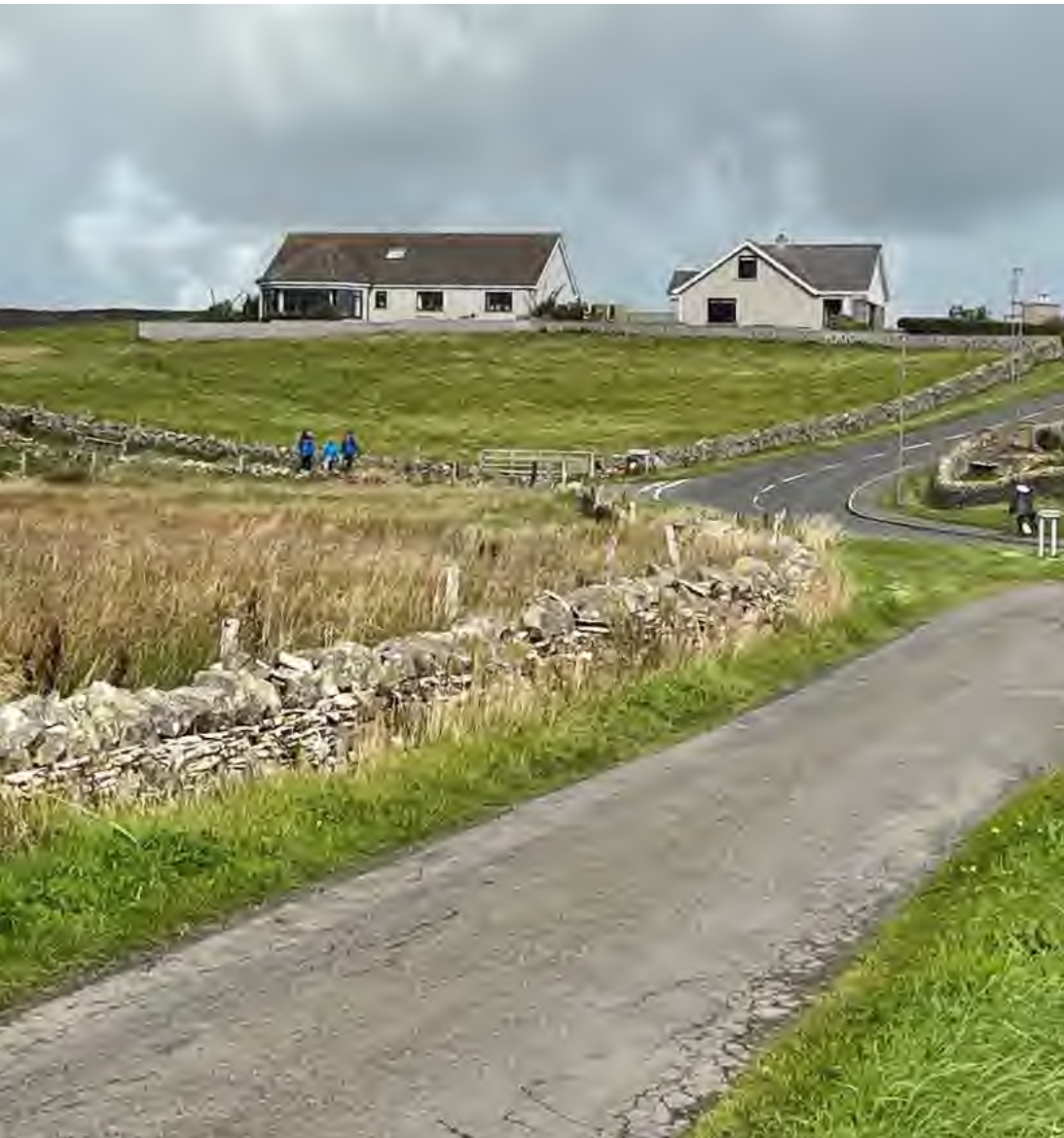
Figure 29: View of Back Road, Nethererton Road and Croval Road junction with lower part of STR-16 visible
