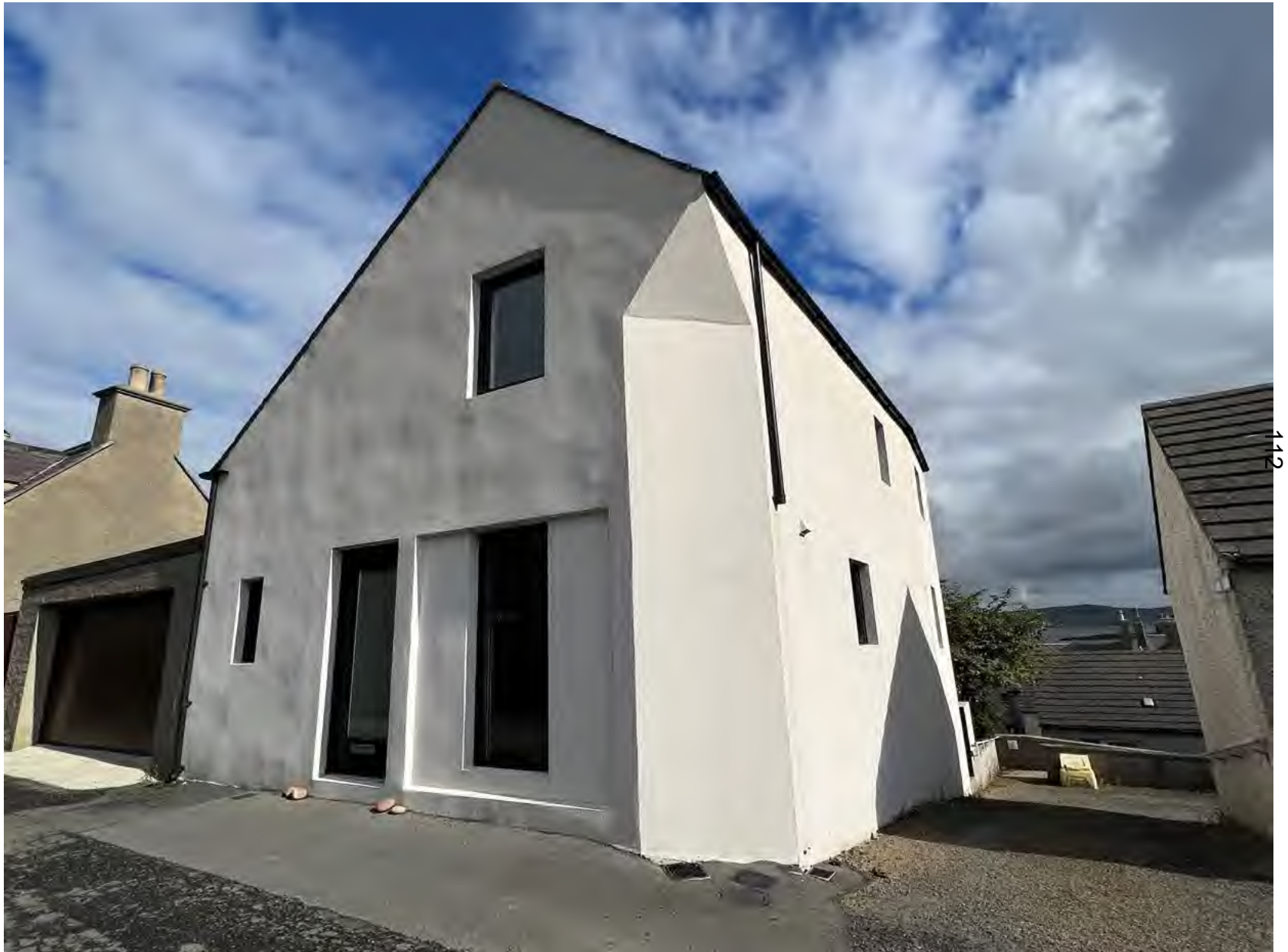
Figure 21: Architectural reference to chamfered corners seen in historic core
