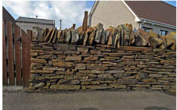
traditional laid dry stone wall
