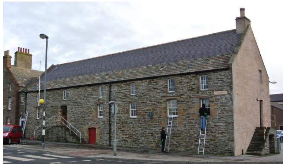
Above: The Girnel on Harbour Street, which is roofed with a combination of Welsh slate and sandstone tiles
