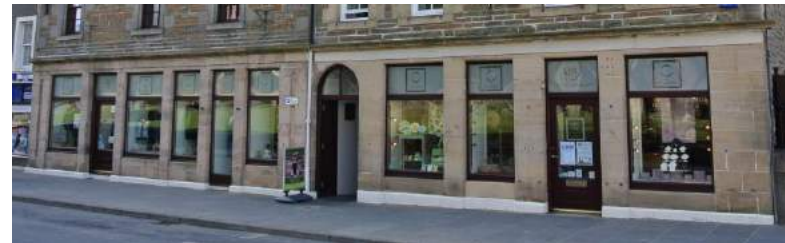
Stone shopfront at 7-15 Broad Street
