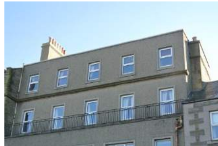
Cement render on the extension to the Kirkwall Hotel
