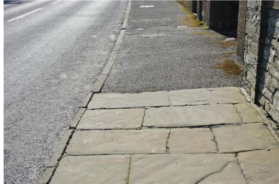
Historic and modern pavement surfaces and kerbs on Dundas Crescent
