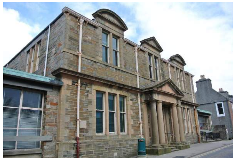
Former library on Laing Street
