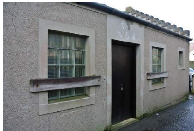
Protective boards for the Ba' over windows on St. Magnus Lane
