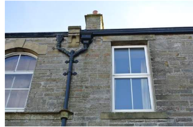
Ornamental downpipes at 16-18 Harbour Street
