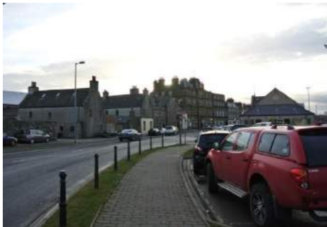
The approach to the town centre along Shore Street, with Tounigar prominent on the left
