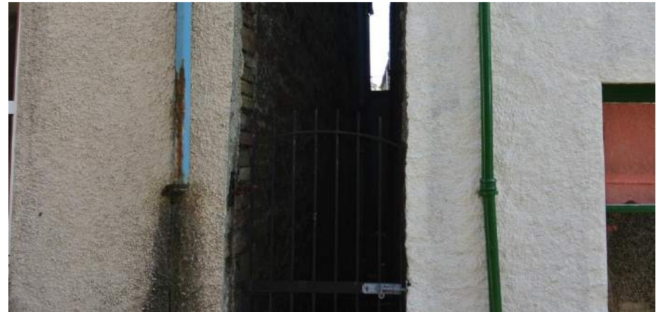
Coloured downpipes on Main Street
