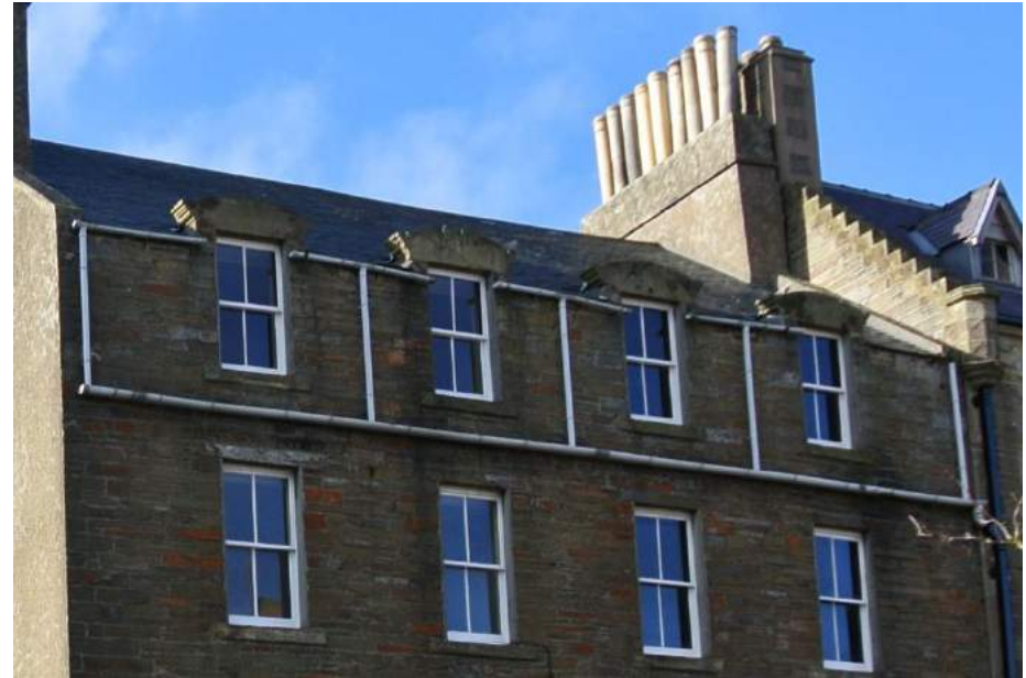
Prominent rainwater goods on Broad Street
