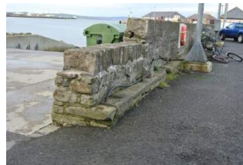
The historic stone wall on the West Pier
