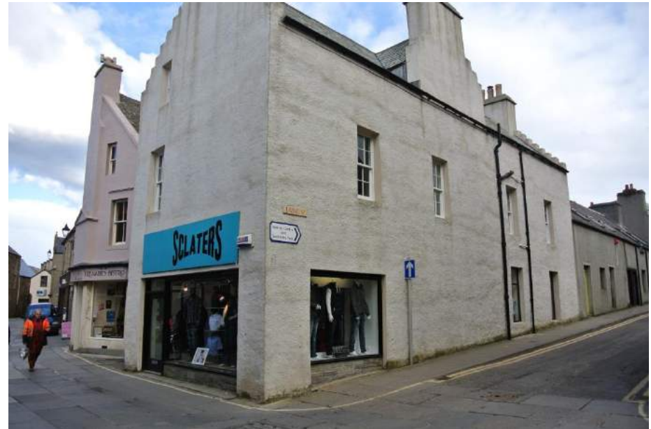
The junction of Albert Street and Laing Street
