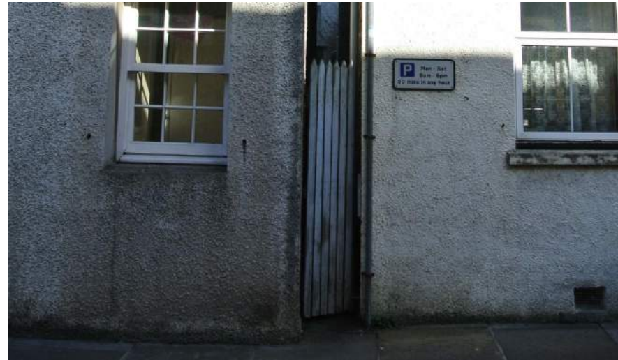
An 'almost adjoining' gap on Victoria Street, blocked by wooden fencing
