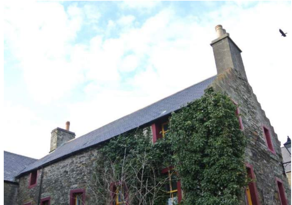
The roof of the Ivy House (43 Albert Street)
