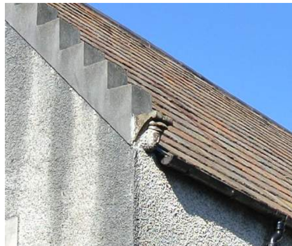
Above: The Girnel on Harbour Street, which is roofed with a combination of Welsh slate and sandstone tiles
