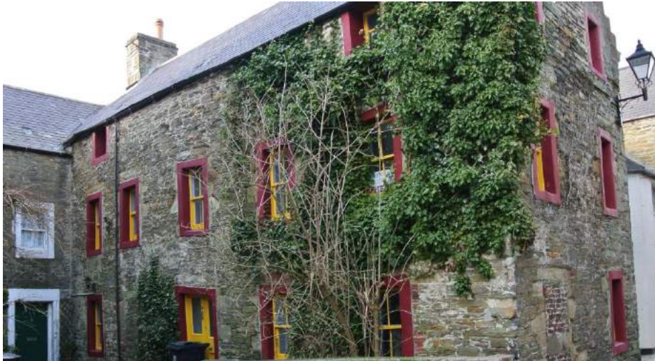
Above: Sash-and-case window on Cromwell Road
