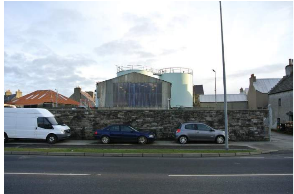
The boundary wall around the fuel depot on Shore Street
