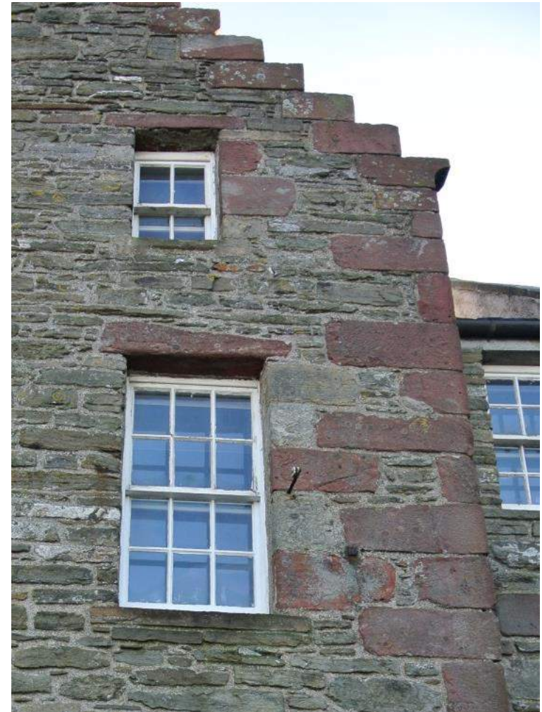
Windows at the Girnel-keeper's house, Harbour Street
