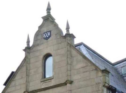
Left: Date stone at 1 Albert Street
