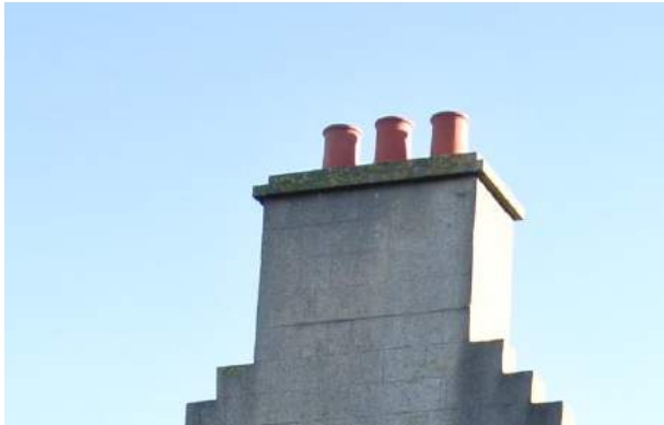
Chimney on Shore Street
