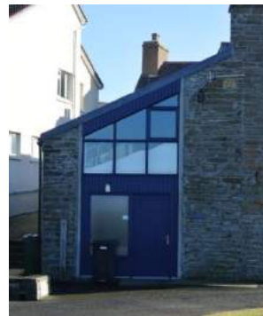
Left: Timber boarding at Dunkirk
