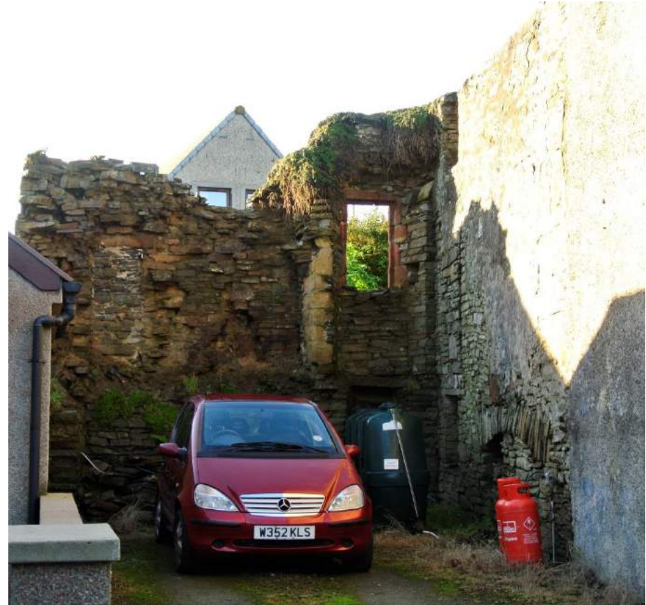
Ruin at the west end of Main Street
