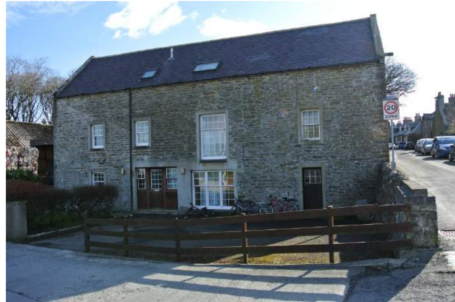
Papdale Mill, Mill Street
