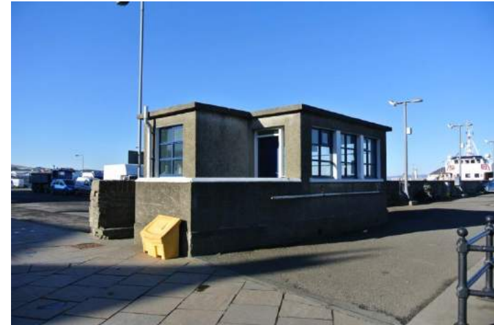
Building at the head of the West Pier
