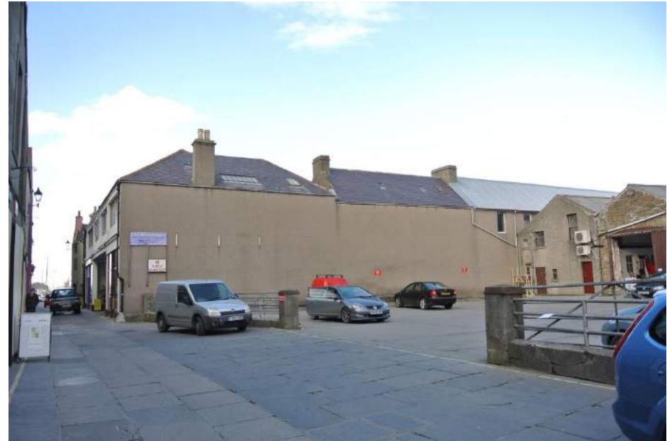
Gap site on Bridge Street
