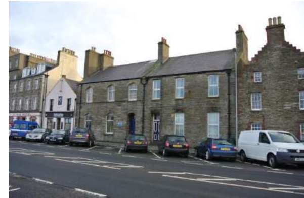
Below: Notes on how 16-18 Harbour Street contributes to the special character of the area
