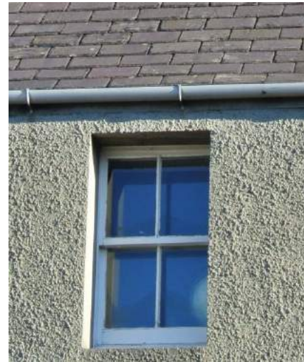
Above: Sash-and-case window on Cromwell Road
