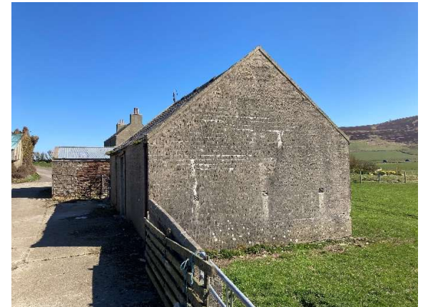
Building 3 (west) candidate for 1 for 1 redundant building
