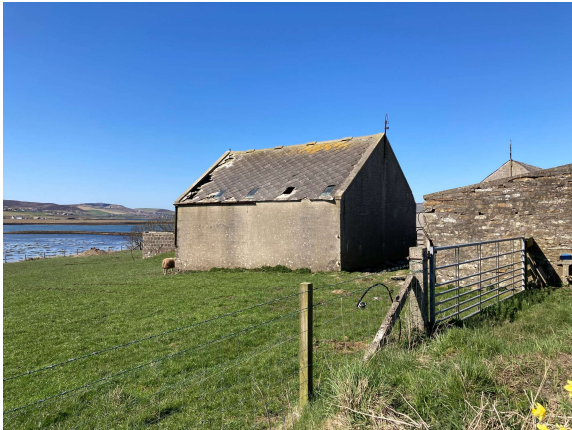
Building 3 (south) candidate for 1 for 1 redundant building
