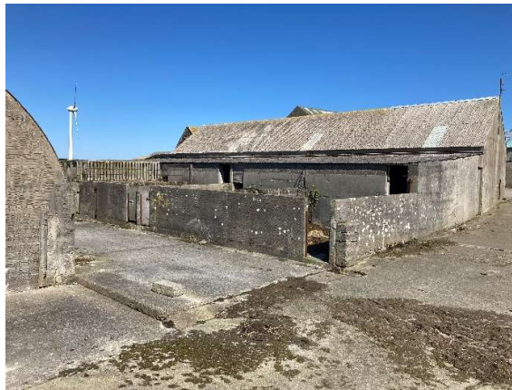
Building 5 and corner of building 6
