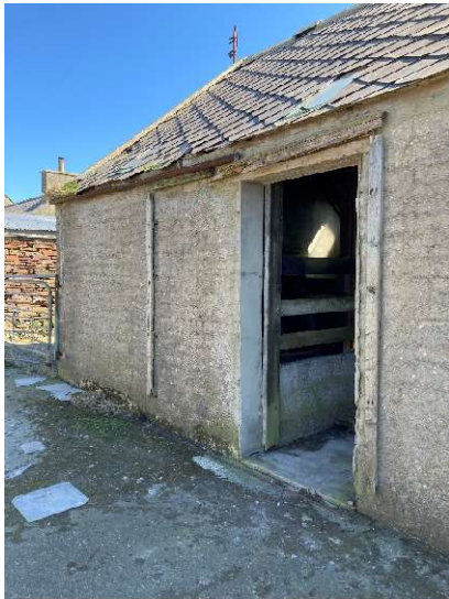
Building 3 – tight/small entrance
