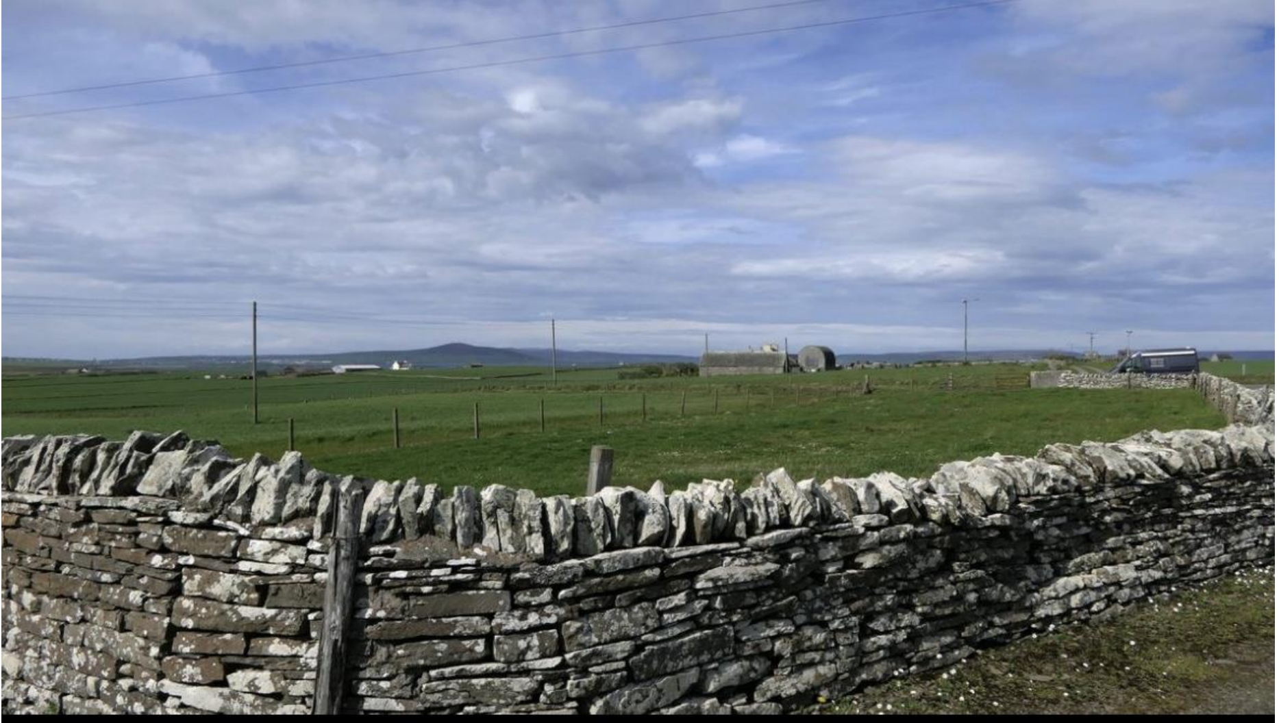
North East Corner
