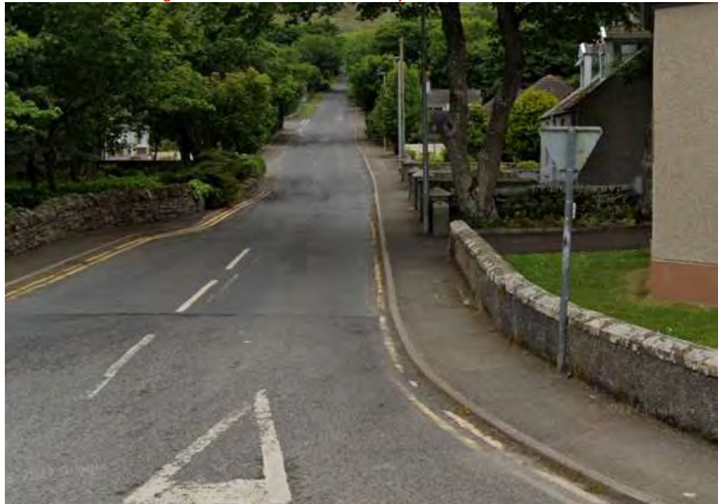
Figure 7. General Standard of Footways on Heddle Road
