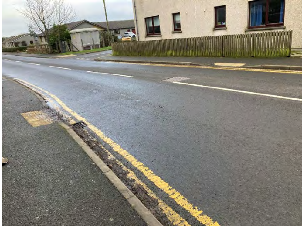
Figure 5. Uncontrolled Crossing Facilities at A965/A966 Junction
