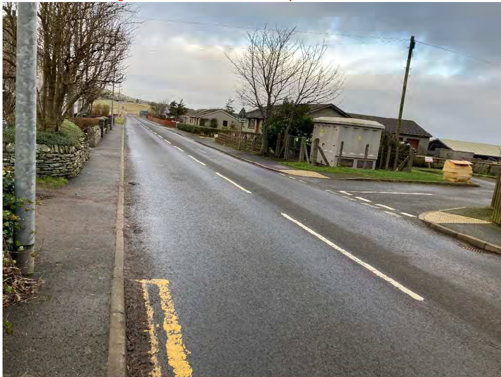
Figure 9. General Standard of Footways on A966
