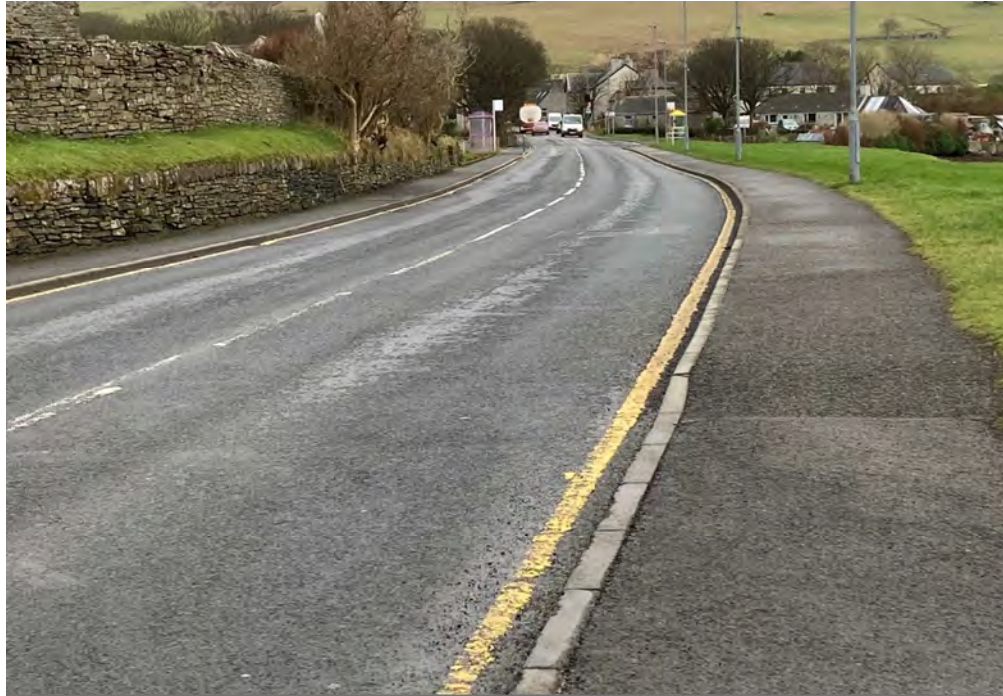
Figure 2. General Standard of Footways on A965
