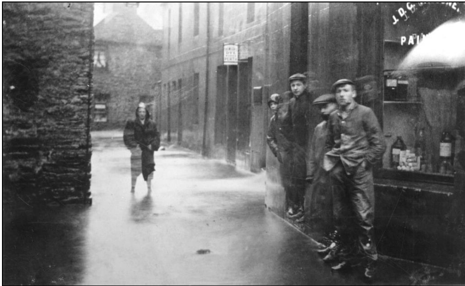
Flooding in Stromness, date unknown, circa 1909.
