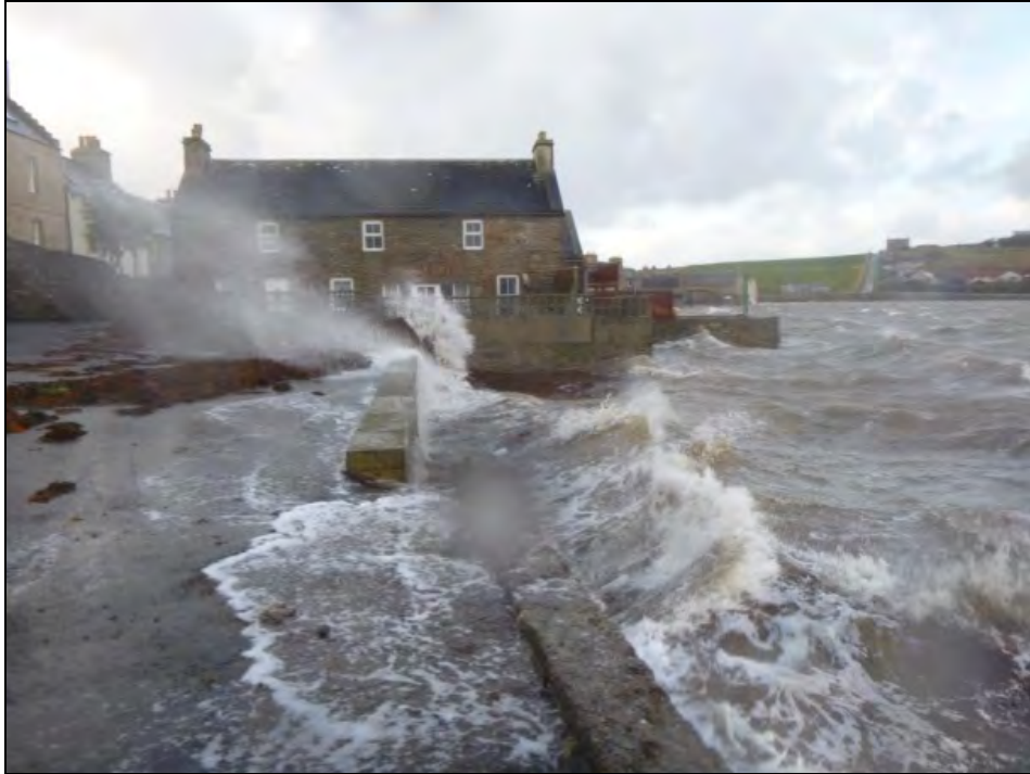
Coastal flooding and wave overtopping, Front Road, St Margarets Hope, 5 December 2013.
