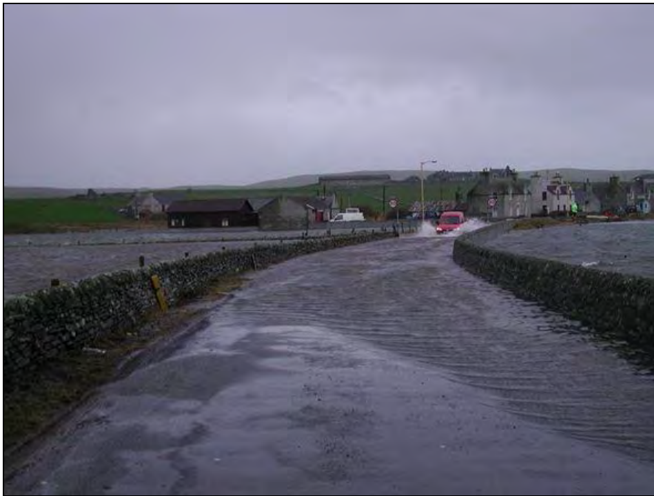
Coastal flooding, Pierowall, 12 January 2005. Photograph courtesy of Danny Harcus.
