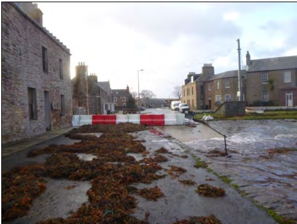
Deployment of mobile flood defence units. Front Road/Cromarty Square, St Margarets Hope, 5 December 2013.
