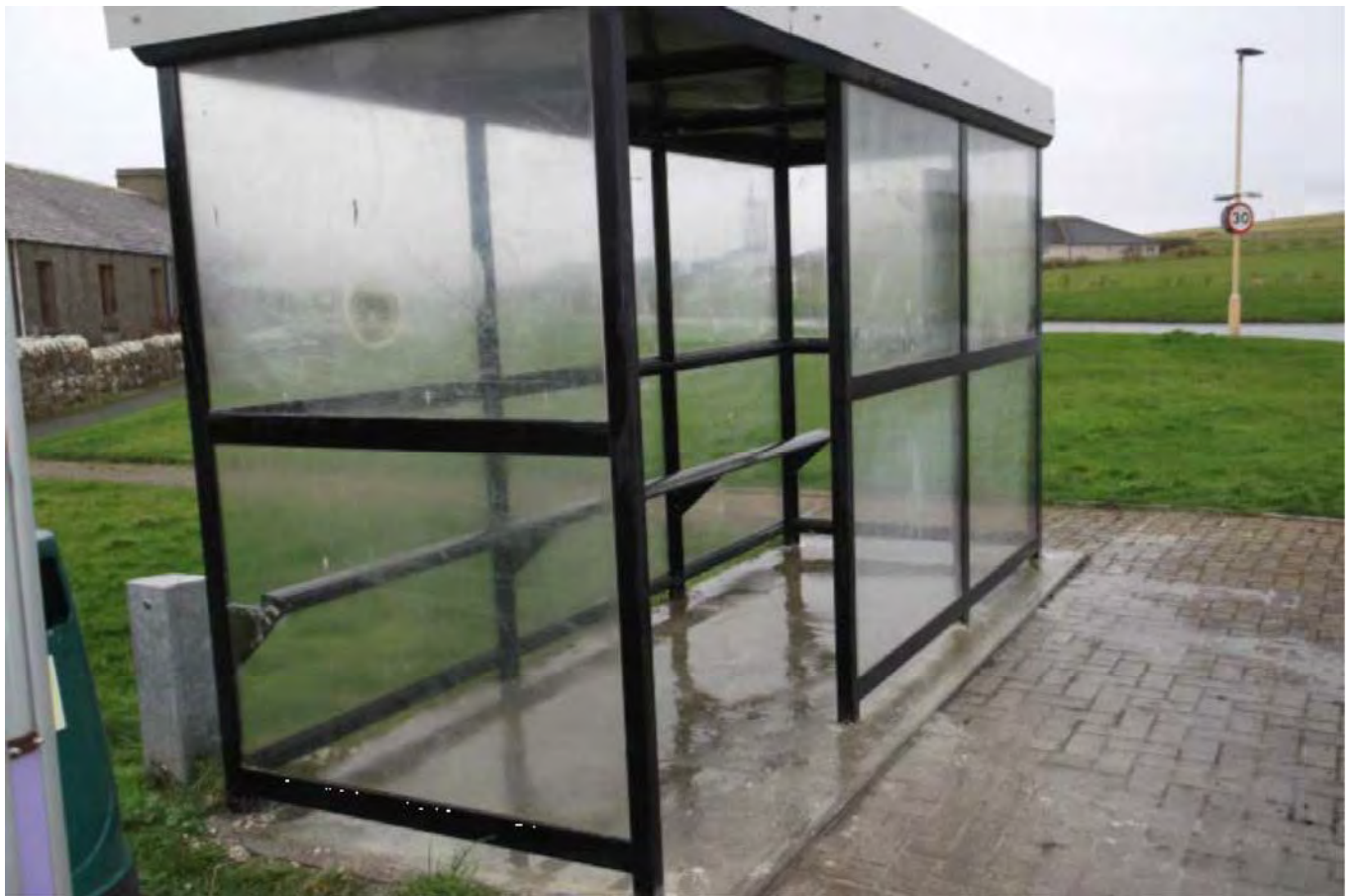
Bus shelter, Burray - After
