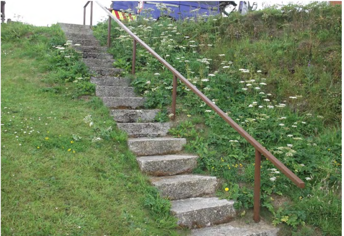
Repainted hand railing, Deerness
