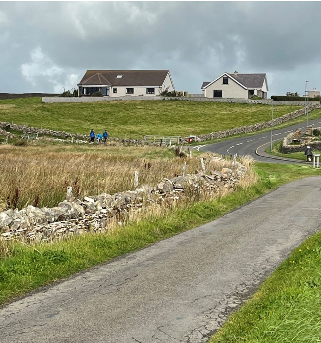
Figure 29: View of Back Road, Netherton Road and Croval Road junction with lower part of STR-16 visible
