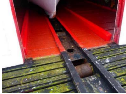
Damaged bottom rails
