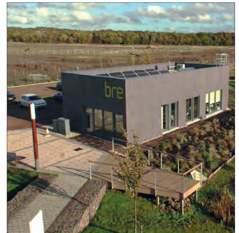
Image of precedent project, BRE Ravenscraig interpretation centre - passive design & pre-fabricated unit
