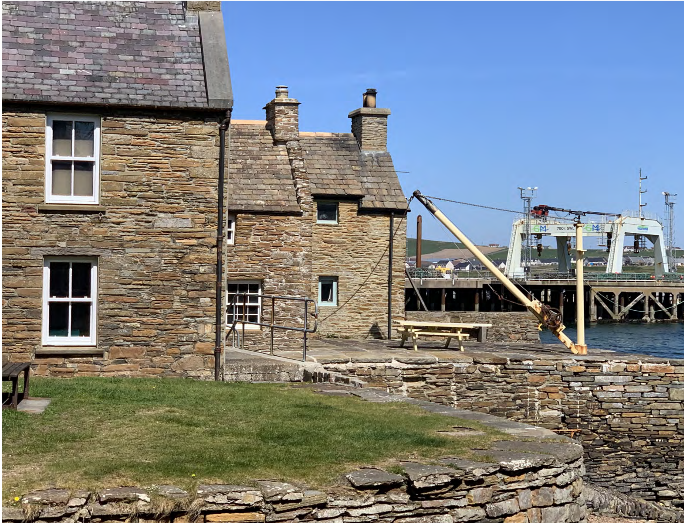
View of piers from Stromness Museum
