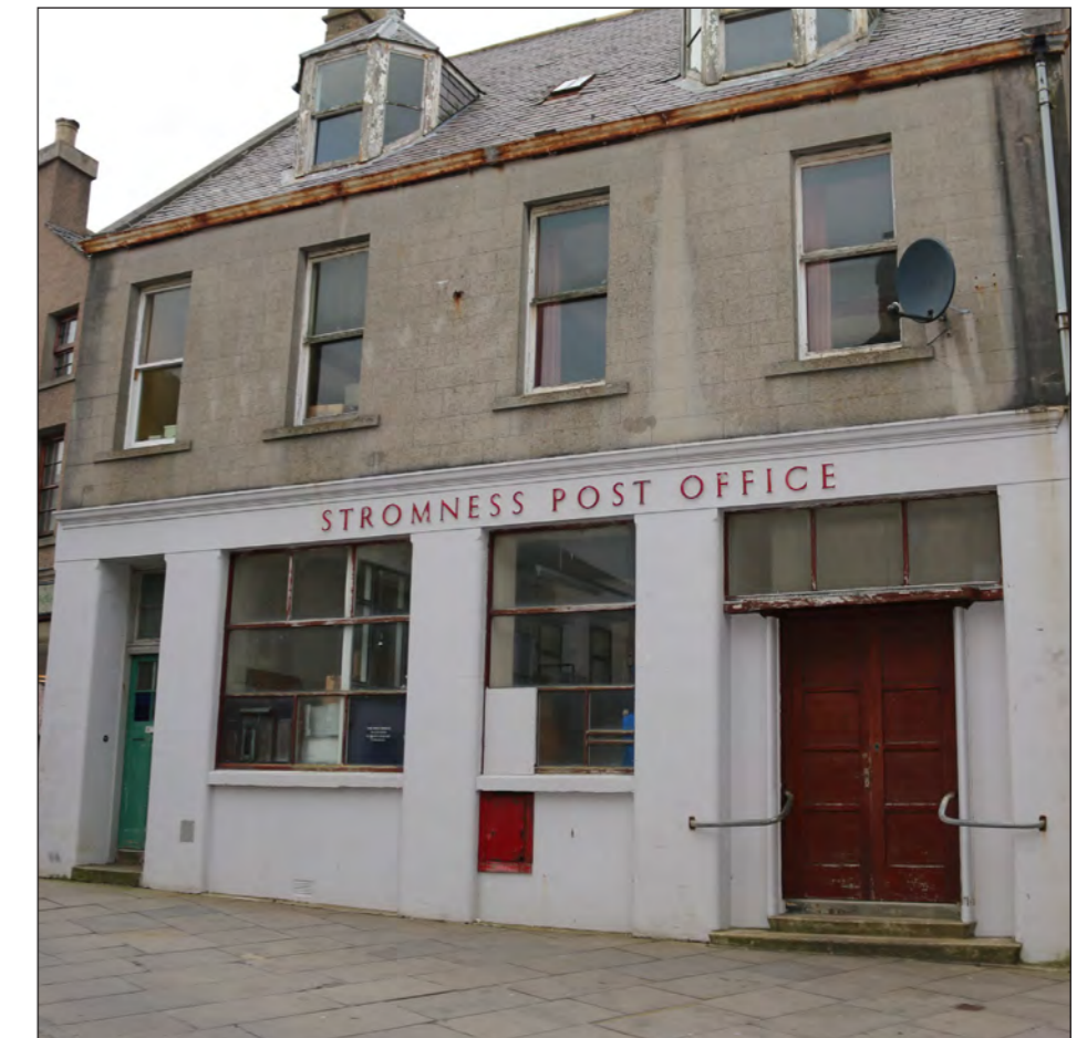
Existing Stromness Post Office
