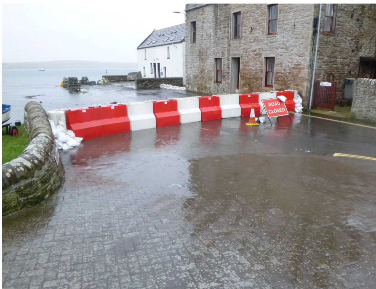
Flood barriers deployed at St Margaret's Hope
